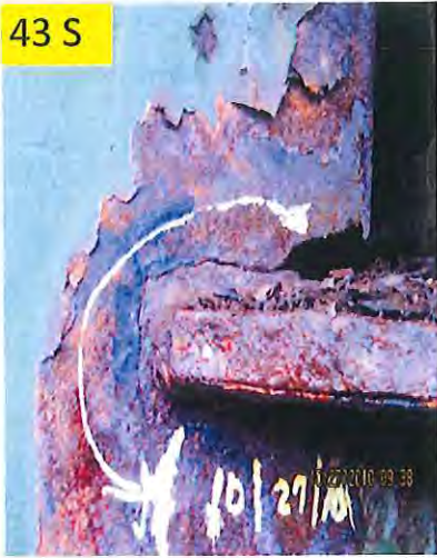
South Seat Area of Span No.2
