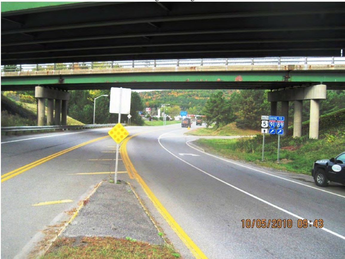
Looking West along US 5
