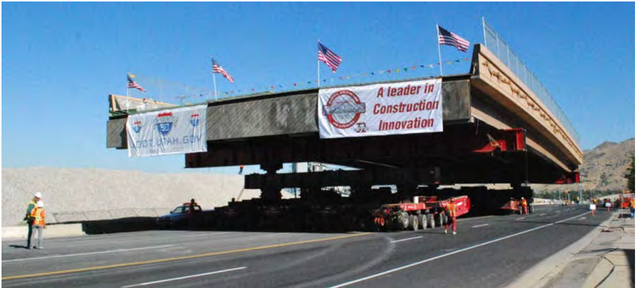
Figure 2: SPMT transporting a bridge superstructure
