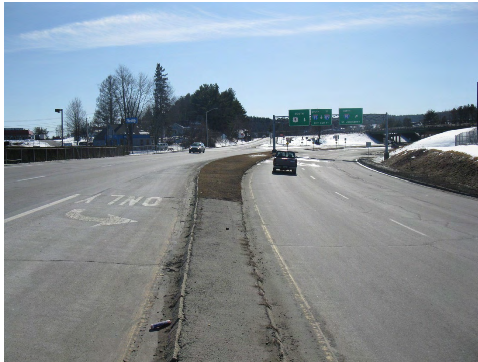
Figure 11 - Route 5 looking westbound toward Ramp D (on right).
