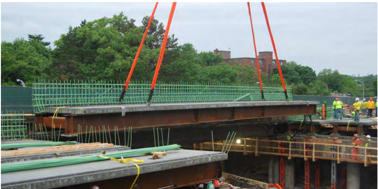
Figure 3: PBU being lifted into place
