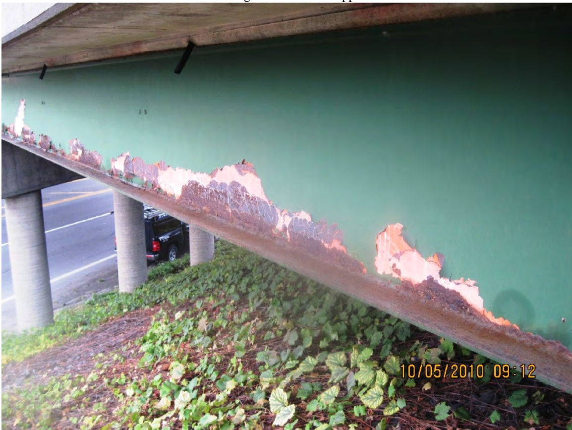
Paint Deterioration
