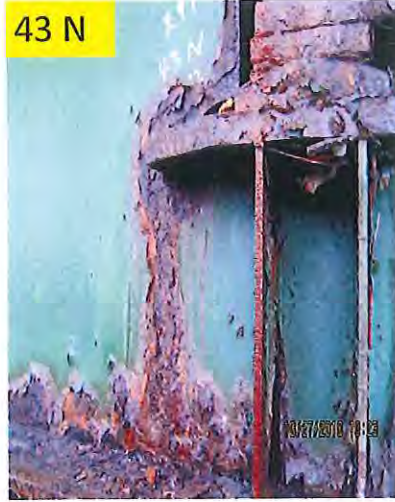
North Seat Area of Span No.2
