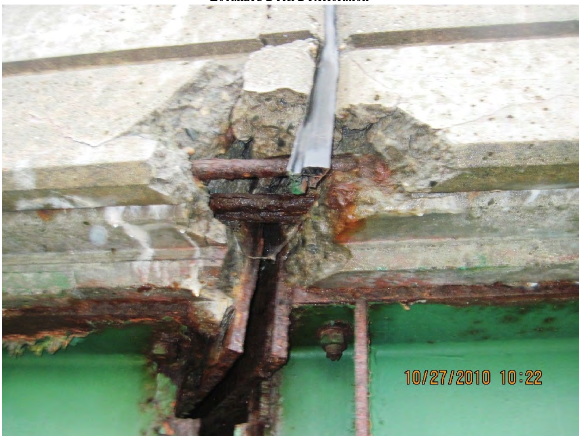
Joint Deterioration
